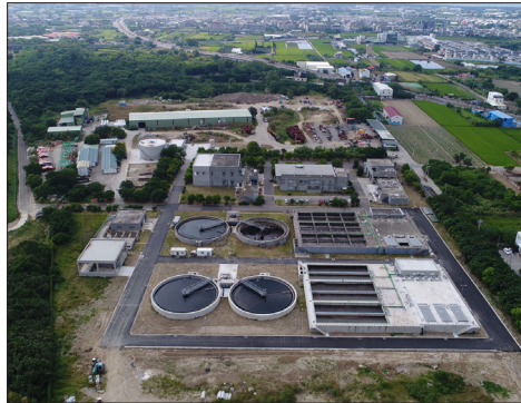
Zhunan Toufen Water Resources Recycling Center
