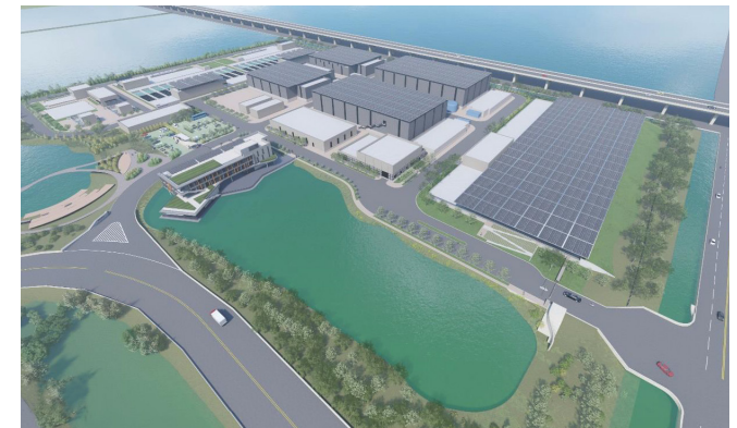
Project of Tainan Seawater Desalination (Aerial View)
