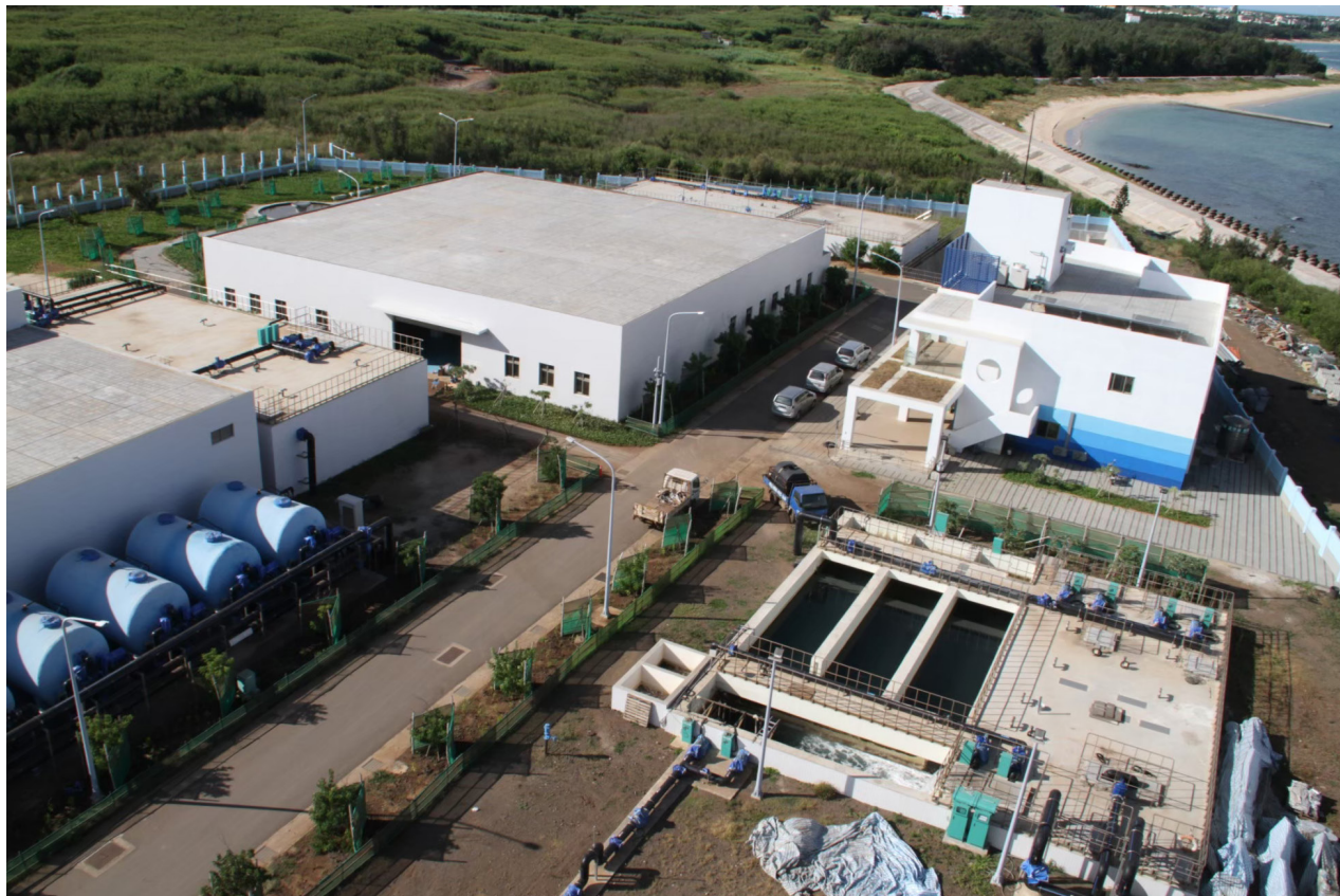
Magong Plant 2 (4000 CMD) Seawater Desalination Plant
