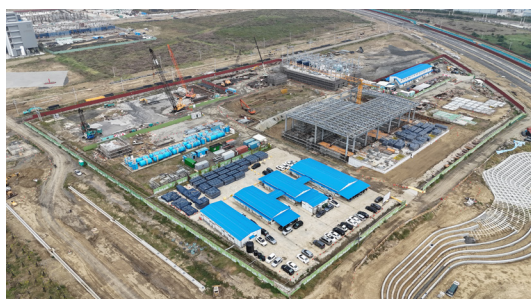
New construction of sewage treatment plant phase I at the Second Kaohsiung Science Park of Southern Taiwan Science Park, South Taiwan Science Park
