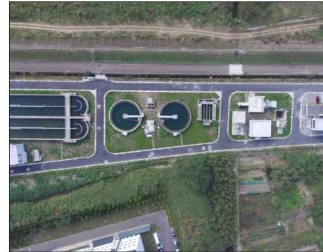
Houlong Water Resources Recycling Center
