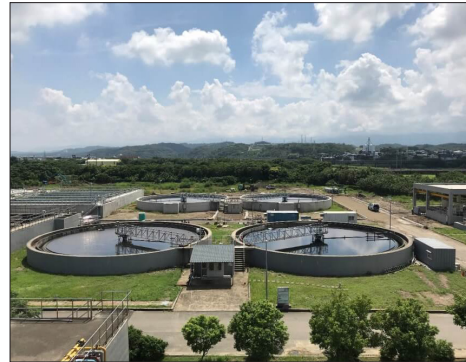
Zhunan Toufen Water Resources Recycling Center (Secondary Clarifier)
