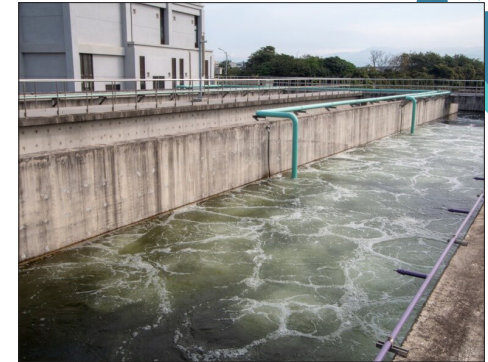
Houlong Water Resources Recycling Center (Oxidation Ditch)
