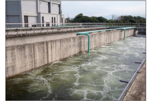
Houlong Water Resource Recovery Center (Oxidation Ditch)
