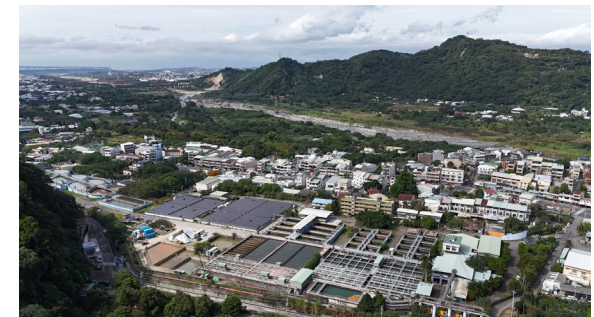
Fengyuan Water Treatment Plant No. 1 Phase I & II Purification Facilities Renewal EPC Contract
