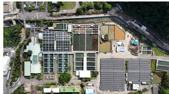
Fengyuan Water Treatment Plant No. 1 Phase I & II Purification Facilities Renewal EPC Contract
