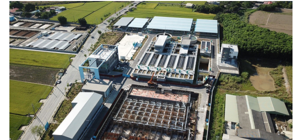
Zengwen Water Treatment Plant Expansion Project – Phase II
