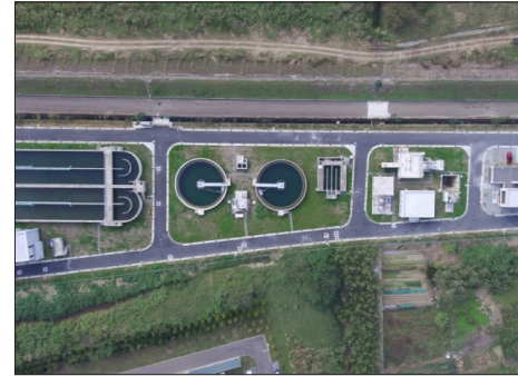
Houlong Water Resource Recovery Center
