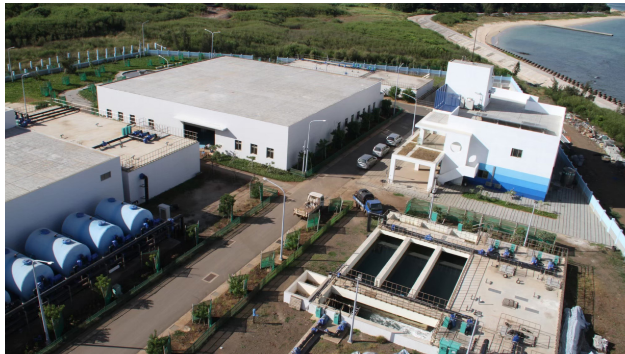
Magong Seawater Desalination Plant II (4,000 CMD)
