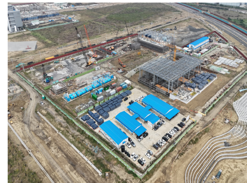
New construction of sewage treatment plant phase I at the Second Kaohsiung Science Park of Southern Taiwan Science Park, South Taiwan Science Park
